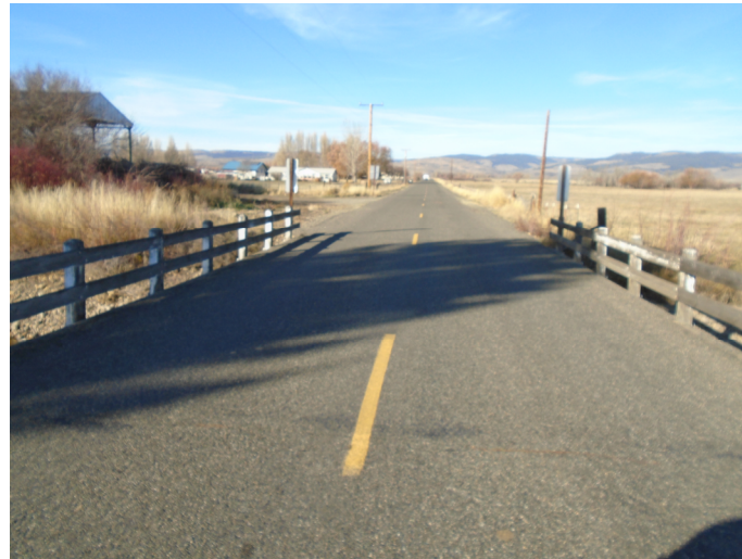
Cooke Canyon Rd looking north
